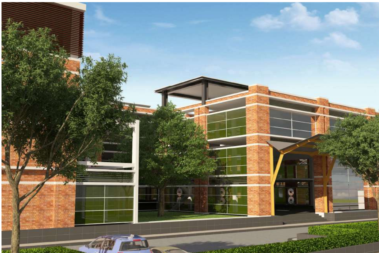
Loading / Unloading Canopy
