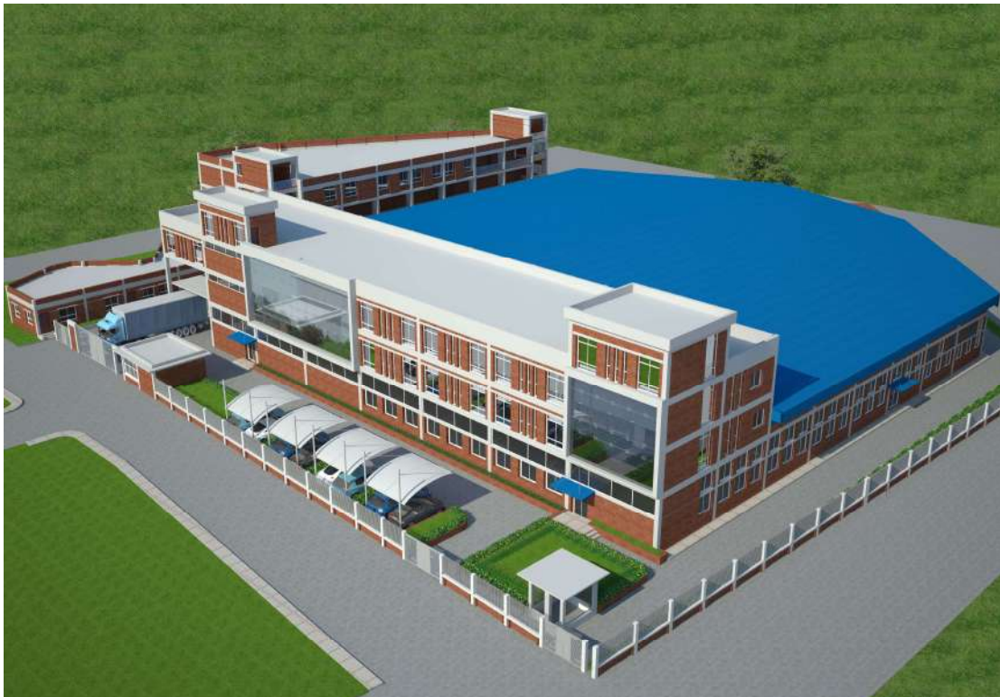
3 storied Garments Building (Sweater Factory)
